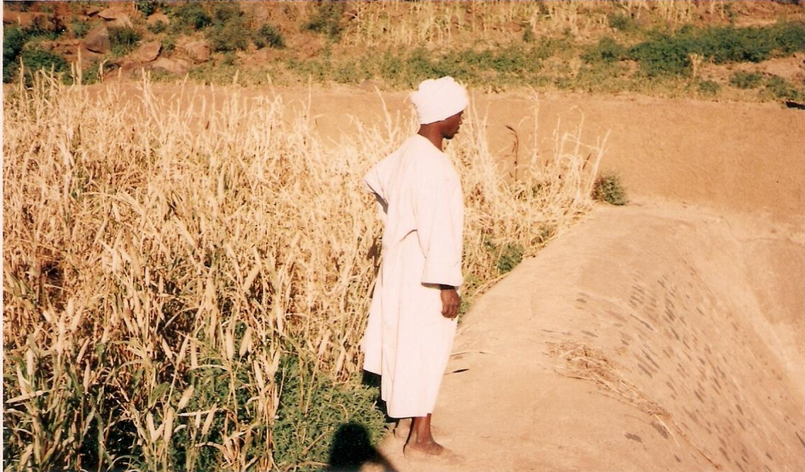
The man is standing on the Golo dam, and the storage area was silted completely and cultivated by Millet (2001)
